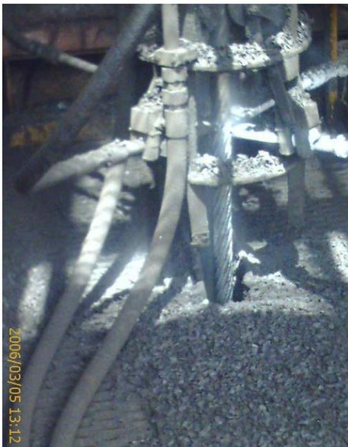
**Figure 7:** Dry ice cleaning removing backfill.
